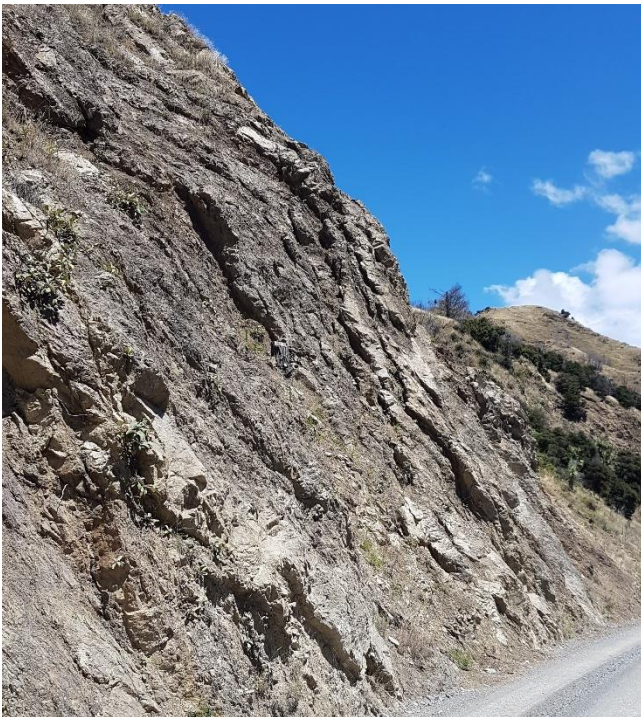
Figure 7: Folded and sheared bedding exposed in the road cuts on Awatere Valley Road.
