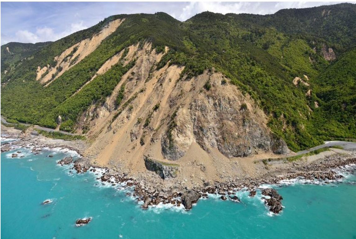
Figure 1. Landslide debris generated by the Kaikoura earthquake, blocking SH1
